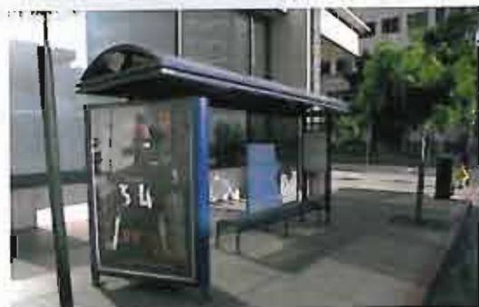
A bus shelter
